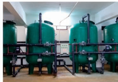
○ 80 m 3 /h过滤设备 80m 3 /h Filter device
