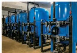
○ 50 m³/h除铁锰设备 50m³/h Iron and manganese removal device
